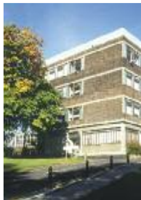
Crawford Theatre, University of Strathclyde, Scotland The roof was prohibited from being subjected to additional loading. The use of the Kingspan KoolDuct® System reduced the overall service loading, and the consequent design strength (and hence cost) of the steel support system.
